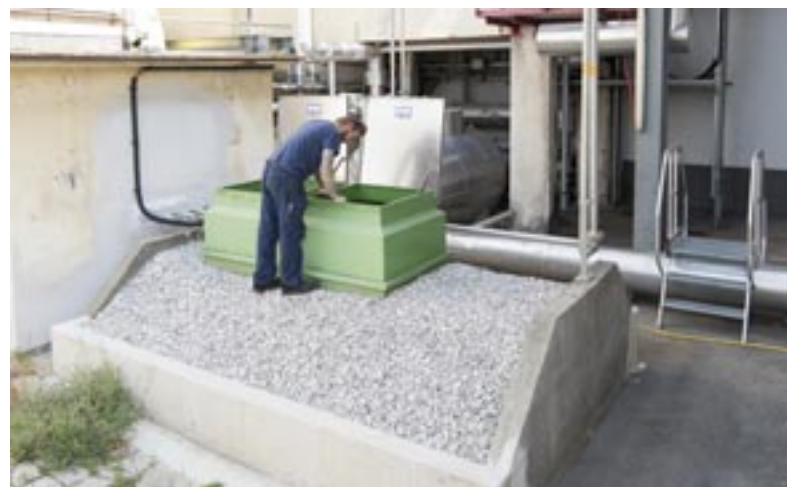
Harald Stassler inspects a manhole shaft (underground solvent tank)
