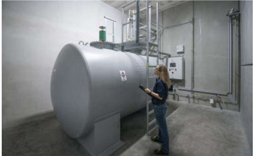
In-process fluids tank with double jacket and leak detector housed in a separate fire compartment
